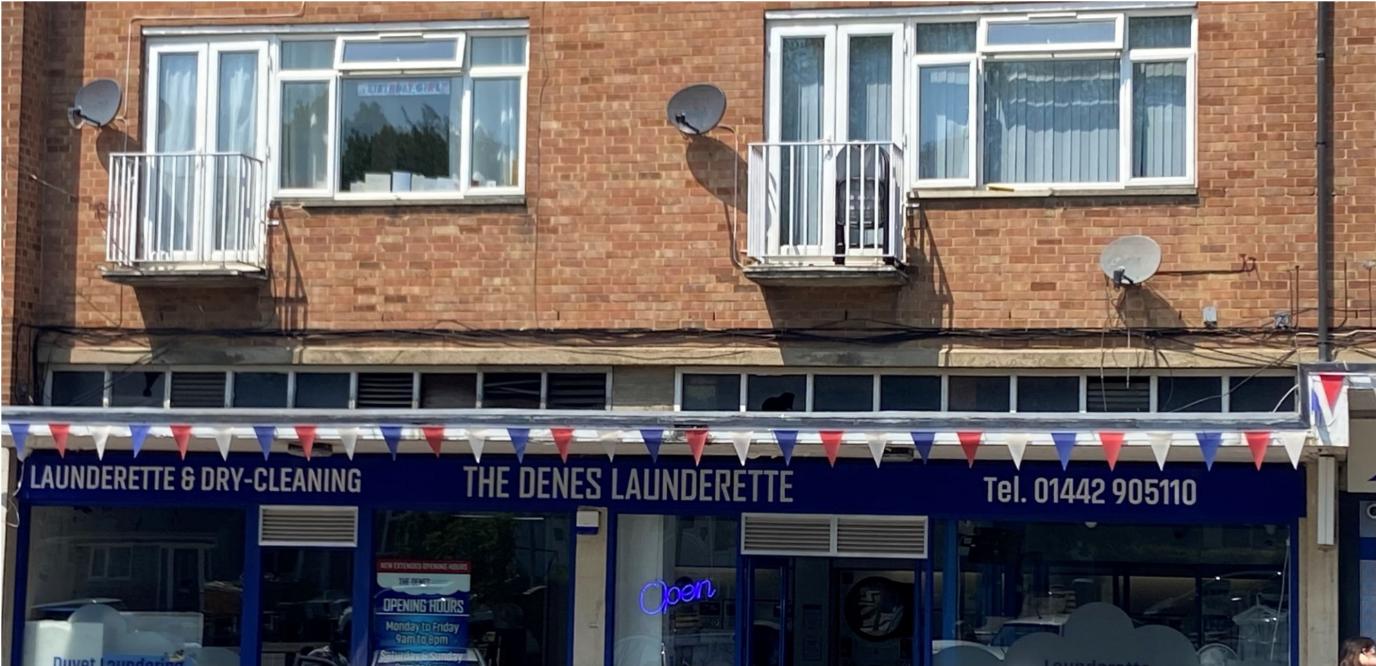
Damaged windows @ The Denes
